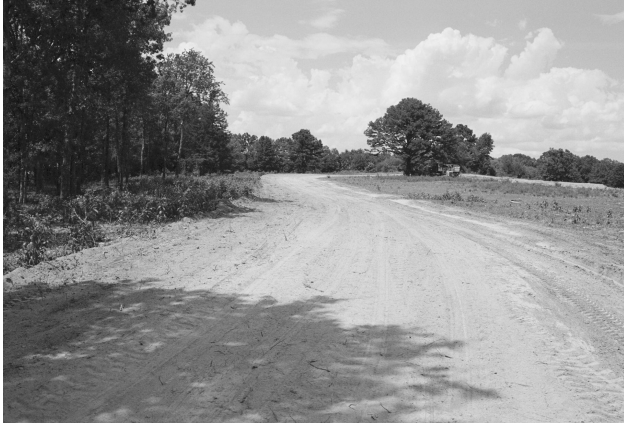
The road to the concession stand. The concession will be built under the large tree with an adjoining picnic area.
